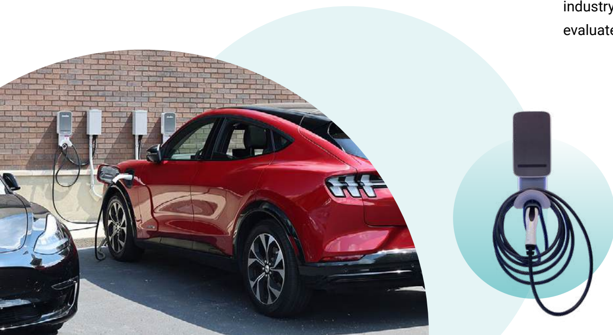
EV Charging Stations at HQ
